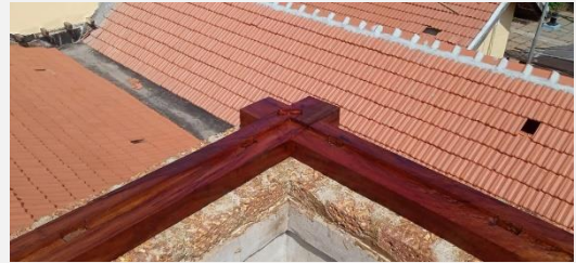
Rañjala wood wall plates fixed
