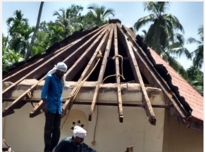
Dismantling of roof in progress
