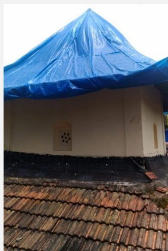
Roof being covered with tarpaulin to prevent leakage of rain water
