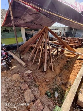
Roof structure assembled at Mahālasā Kalā Kendra, Kumṭā
