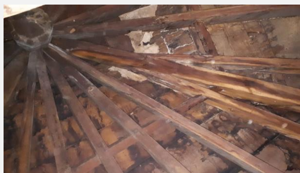
Existing roof which was damaged by termites and dampness.
