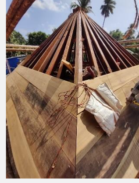
Fixing of Champā wood Planks
