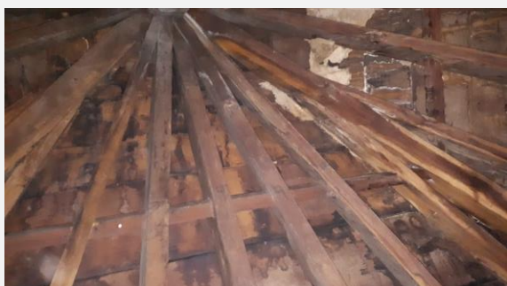
Existing roof which was damaged by termites and dampness.
