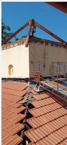
Fixing of Corner rafters and Buruḍe
