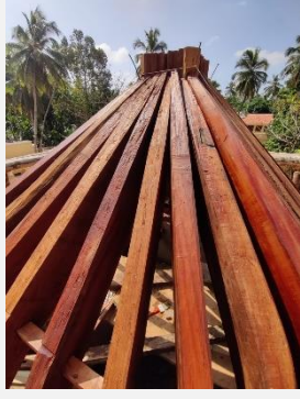
Fixing of all rafters
