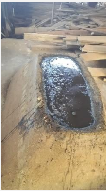
Gāre mortar prepared at Gokaṛṇa and left for fermentation
