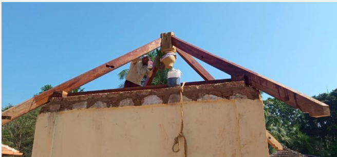
Fixing of Corner rafters and Buruḍe
