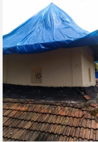
Roof being covered with tarpaulin to prevent leakage of rain water
