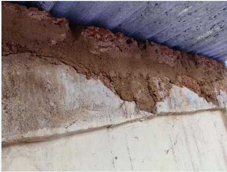
Laterite stone built with Gāre mortar
