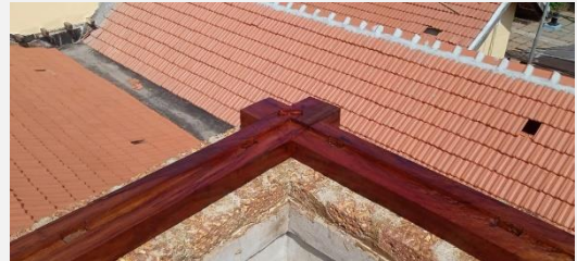
Rañjala wood wall plates fixed
