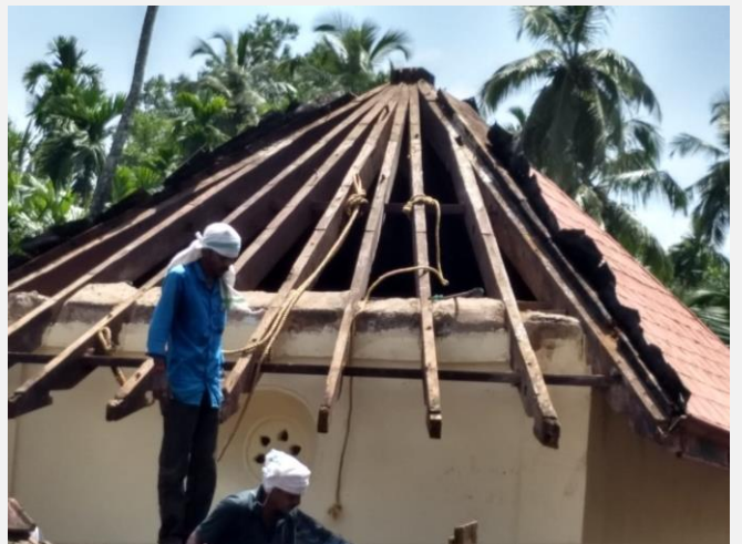
Dismantling of roof in progress
