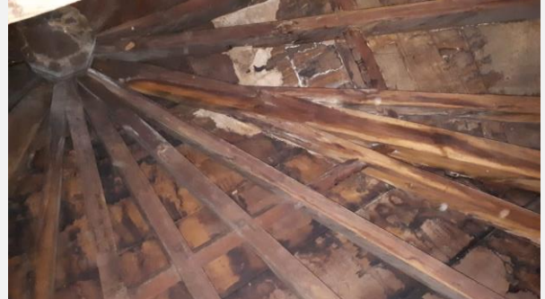
Existing roof which was damaged by termites and dampness.
