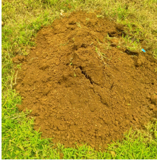
Final closure of the composting pit using the mud excavated while digging the pit.
